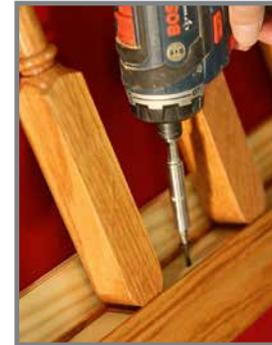
9. Locate the predrilled hole on the flat side of the center of the Shoe Rail. Fasten a screw in there as well.
