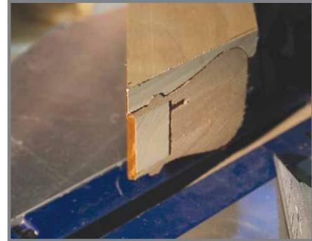
10. Align the entire Amazing Rail™ section between the newel posts (or wall). Make sure the Balusters are plumb with the newel posts (or wall).
