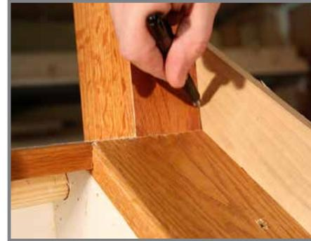
4. Cut the Moulds along the penciled-angles using a Mitre Saw.
