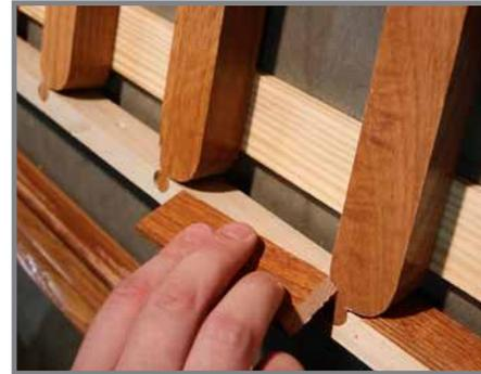
6. After all Fillets have been placed, fit the Inserts (with the fitted Baluster) into their respective Rails by pressing them in firmly.
