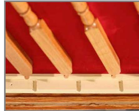
4. Once the Balusters have been set correctly between the Inserts and at an angle, fit the round dowels at the ends of the Balusters into the Insert.
